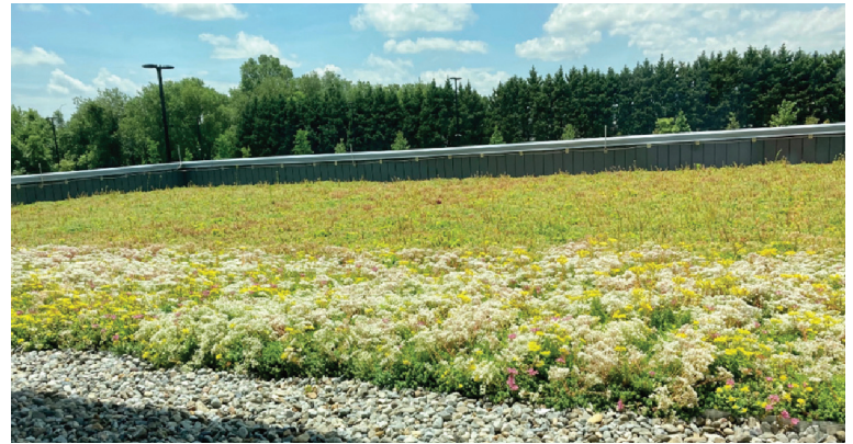
Project: Chesapeake Utility, Dover, Delaware, Photo by: Autumn Chalabala, Chesapeake Utility Director
