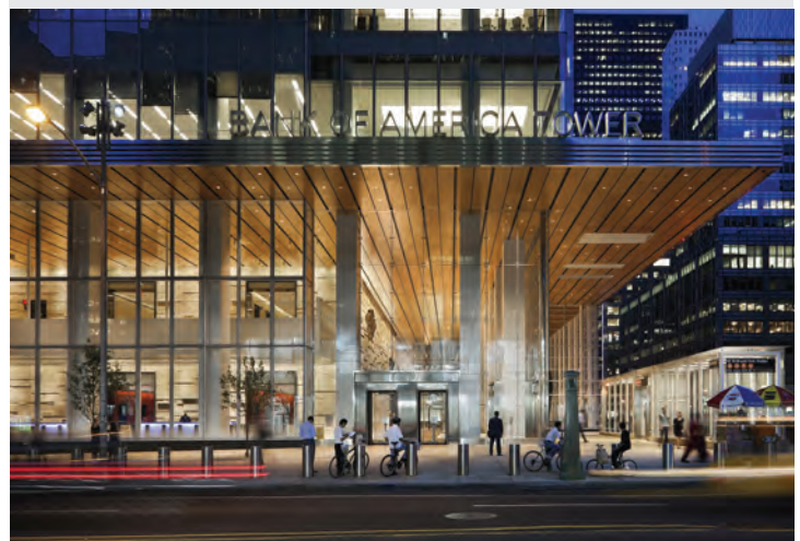
Bank of America Tower in NYC was the first skyscraper to be LEED Platinum-certified. The building uses combined heat and power to provide approximately 65 percent of building’s annual electricity requirements.
